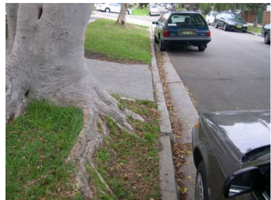
Image 9: Damage to kerb caused by a Hills Fig street tree.
