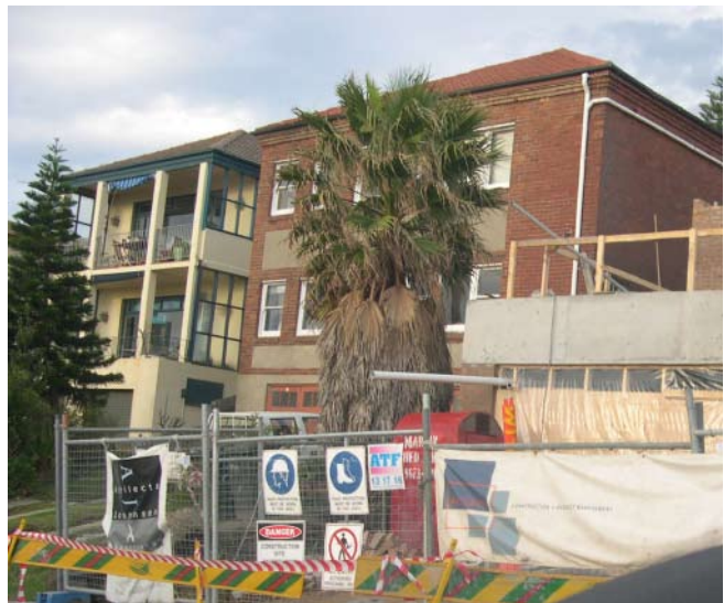
Image 24: Typical tree on a development site in Bondi, requiring protection.
